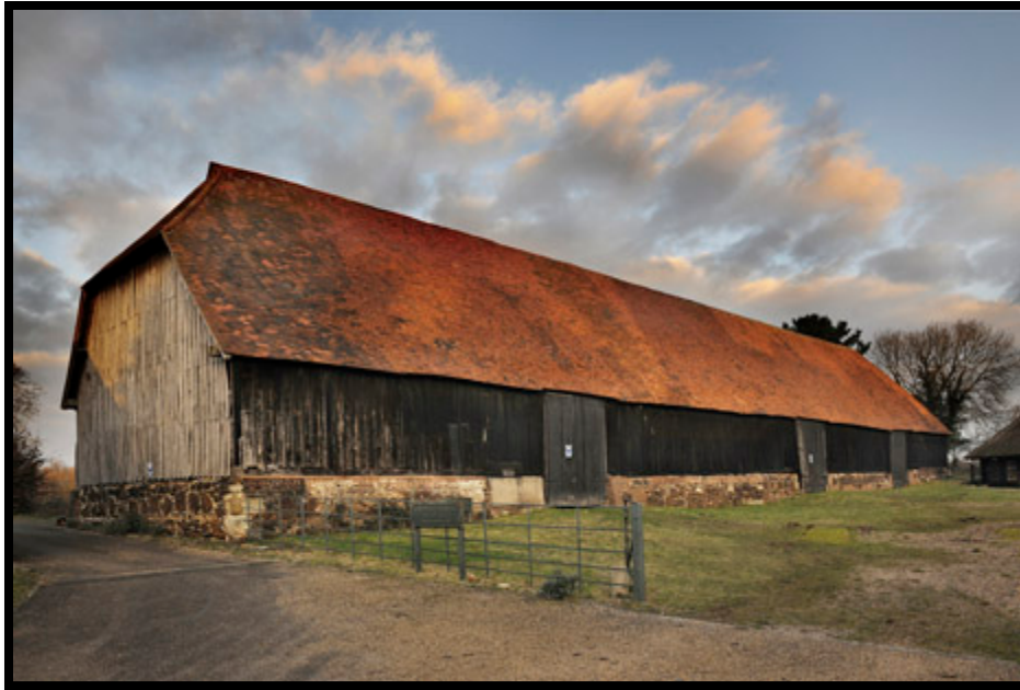
Figure 33: A view of Harmondsworth Barn from the south east. Image from English Heritage
