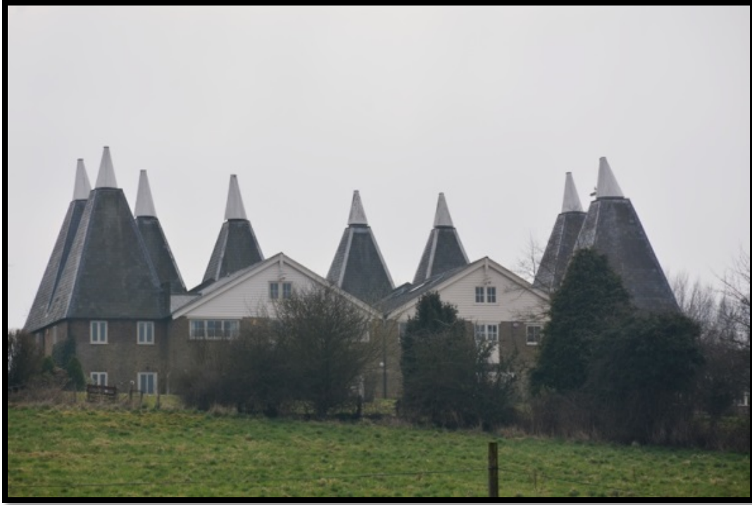
Figure 7: This large complex of oast houses near Maidstone has undergone a domestic conversion.
